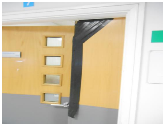
Picture 2: Damaged door
